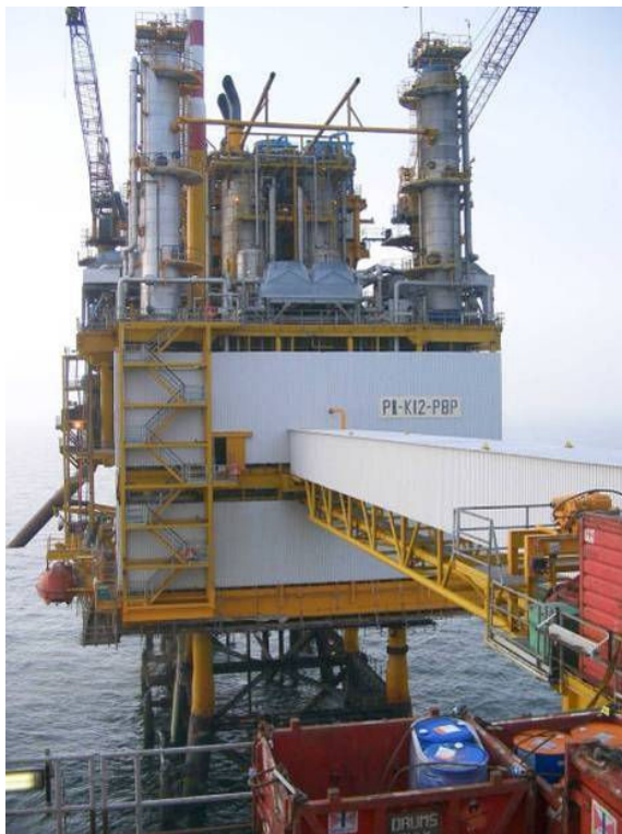
Figure 3: main platform K12-B
