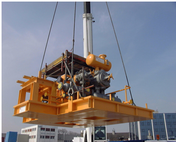
Figure 6: Compressor ready to transfer to K12-B platform
